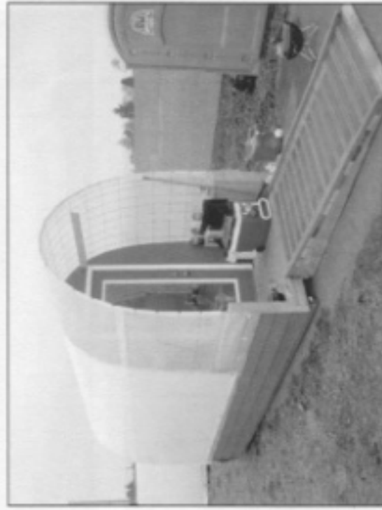
Figure 3. A ramp for use by someone in a wheelchair. Also, notice the Hut is a custom size to accommodate the larger sized door (36") and larger interior space to maneuver a wheelchair.
