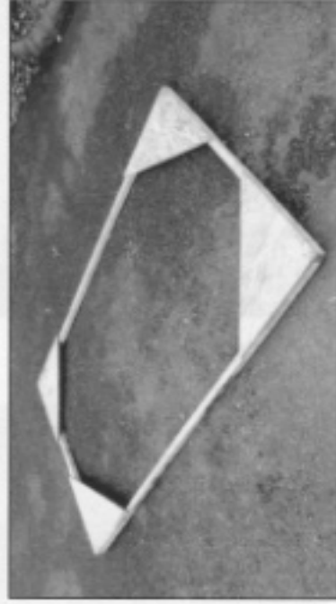
Figure 2. A completed foundation block layout jig
