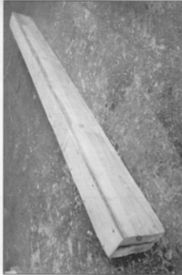
Figure 2. Finished wall footer
