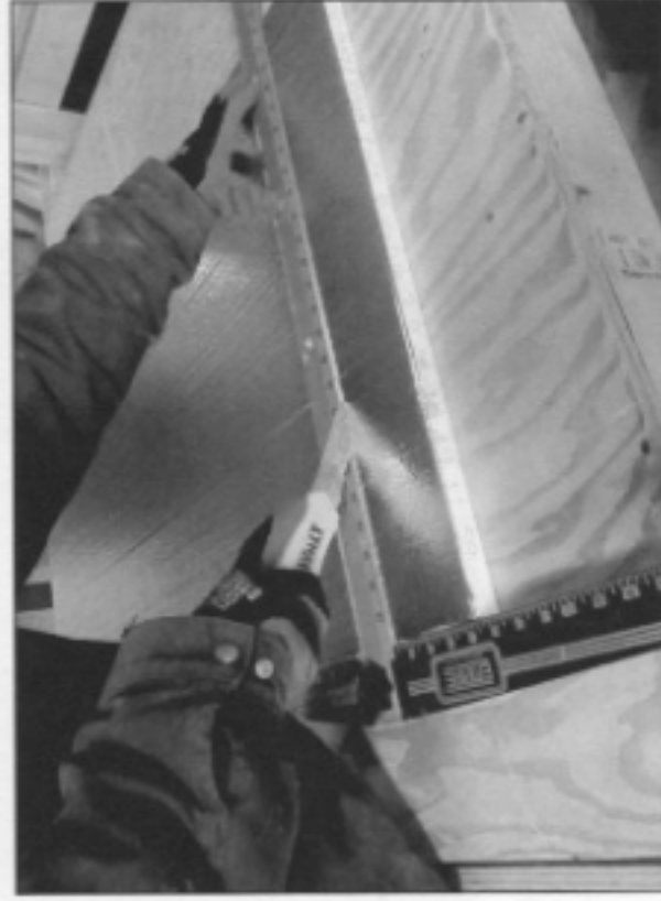
Figure 14. Cut the foam panel with a razor knife with a long blade and a straightedge.
