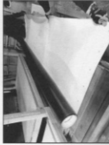
Figure 8. TPO: We purchase pre-cut rolls from a local roofing contractor. Small quantities of TPO are typically not sold at your general building supply stores.
