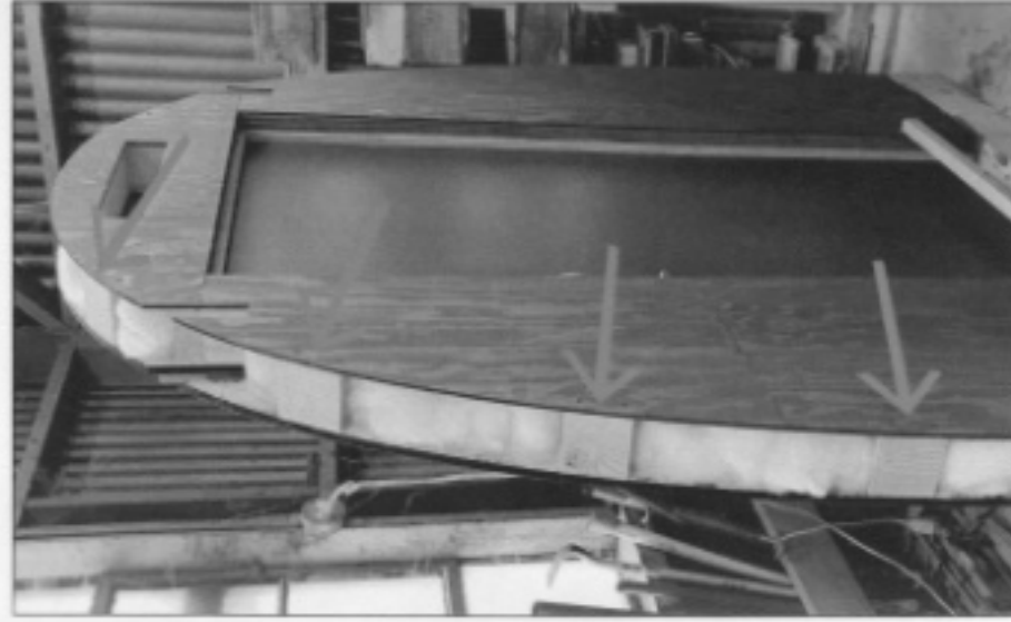
Figure 7. Wall blocks installed
