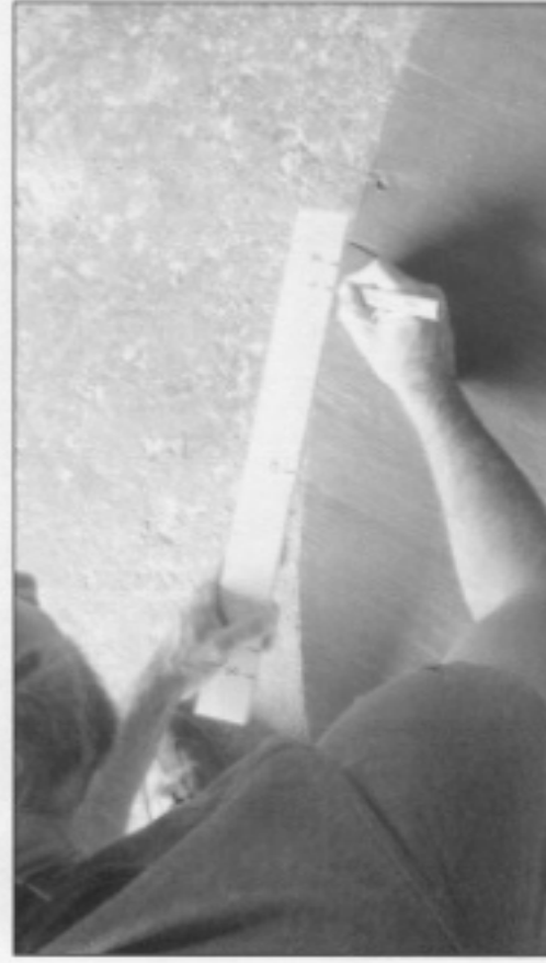
Figure 5. Spacing tool is used to mark the positions of the 2X4 wall blocks.
